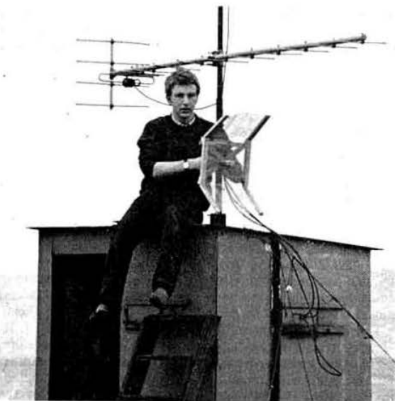
High above the city centre of Bristol, 100 feet above ground level in fact, is this vhf operating centre of G3KAC, belonging to the Bristol University Amateur Radio Society. Adjusting the 23cm trough reflector is G8ADP. Above him is the 14-element aerial used on 70cm, and above that again, out of sight in our picture, is the 8-over-8 which gives G3KAC such a good performance on 2m. The Society owns a TW2 for the 144 MHz band. Frequently this does duty as a drive source for the G8ADP varactor multiplier for 70cm and the 3CX100A5 for 23cm.
